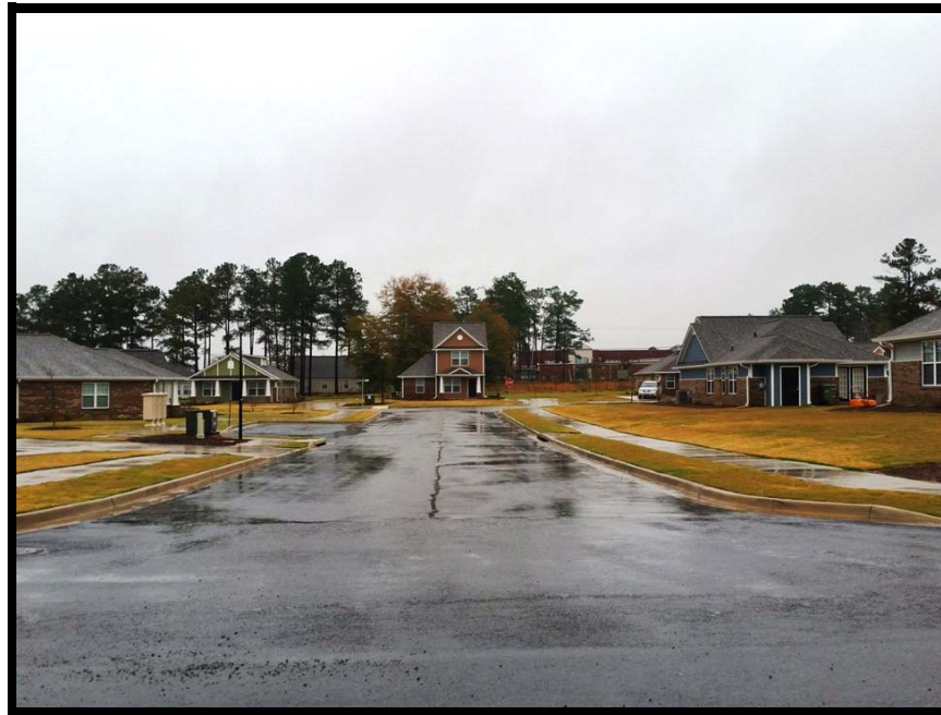
North view from site
