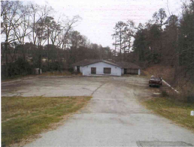
Exiting building on the north end of the site on Lake Murray Boulevard.
