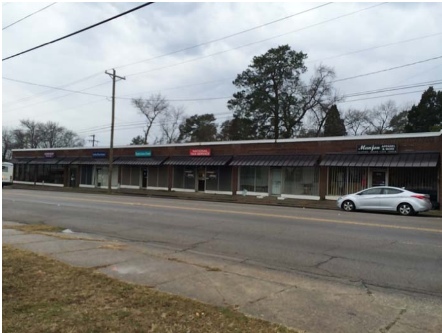
Looking West From Site (Southern End)
