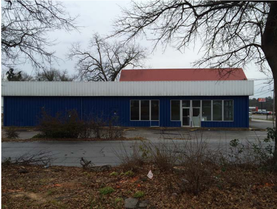
Looking South From Site
