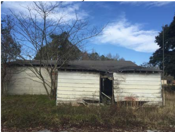
Old structure on site – to be razed
