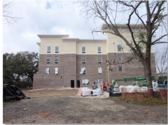
Townplace Suites hotel under construction to the west on Orleans Road.
