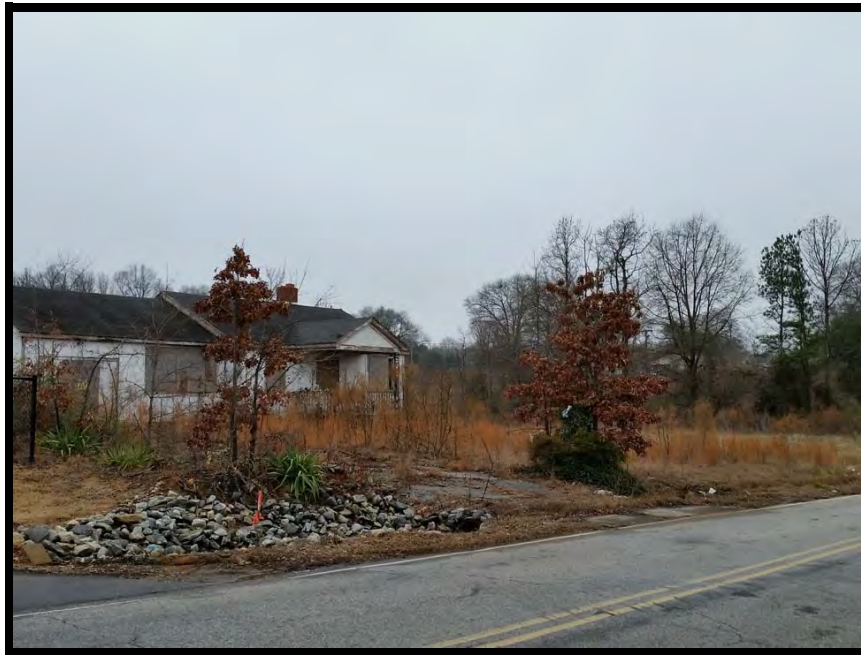
View of site from the northeast
