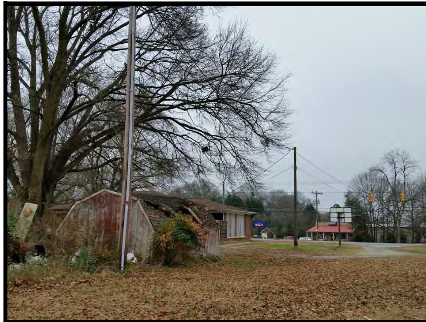
Southwest view from site
