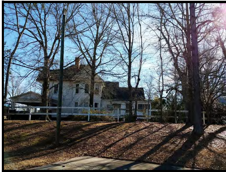
South view from site
