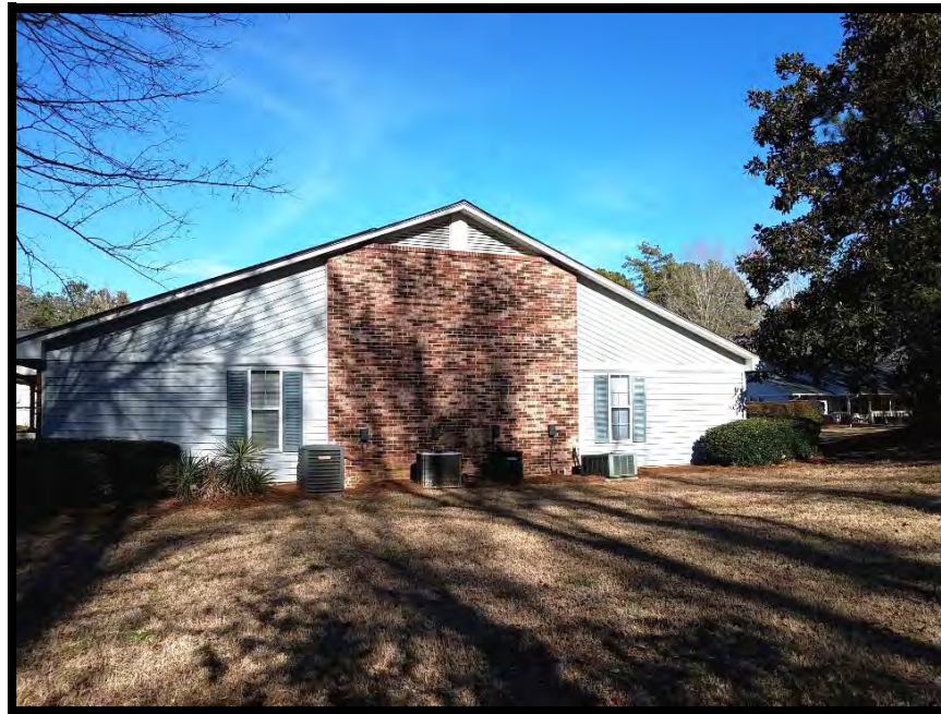
View of site from the southwest
