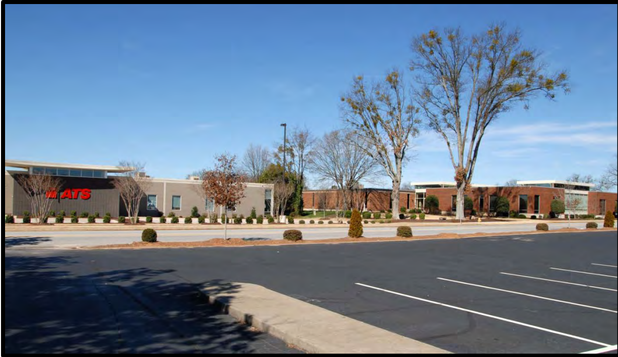
Photo 3—Commercial buildings across Frederick Street. The site is in the foreground.
