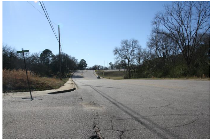
Facing west along Meeting Street Photo taken from Willow Lake Road
