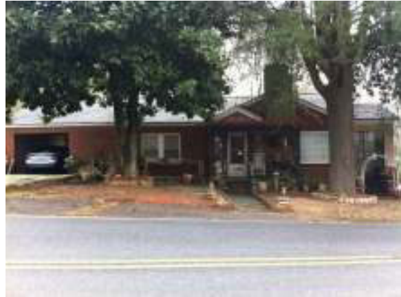
View of a single-family detached home bordering the site to the east
