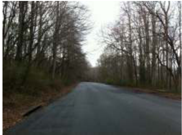
View of Brogan Avenue facing east, site on left
