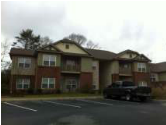
View of Hampton Crest / Greene just east of the site
