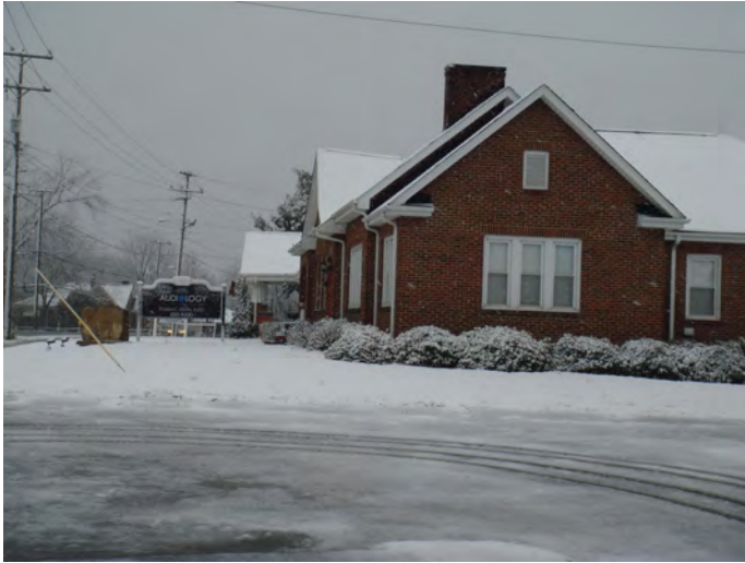
Professional office building on the East side of Site on West Poinsett Street at Oakland Avenue.
