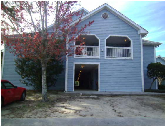
View of end of building wing with staircase.
