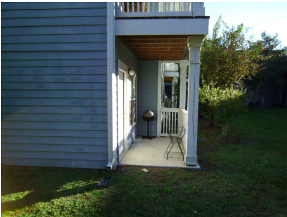
View of patio at rear of building.
