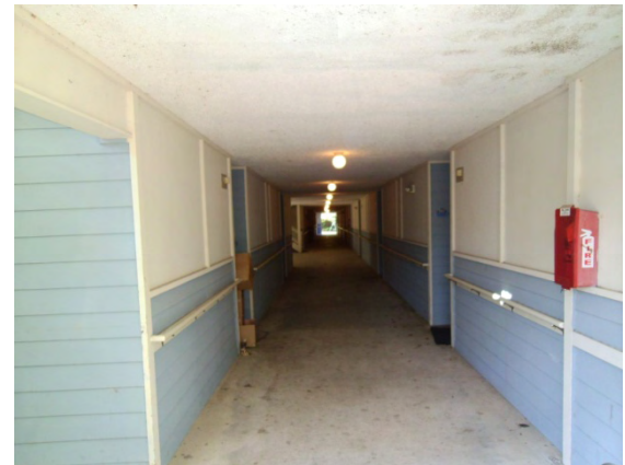
View of corridor on residential wings.
