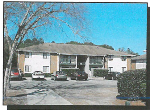
(6) Hillcrest building, south to north.
