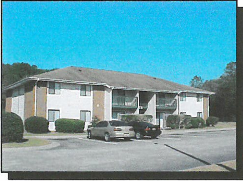
(7) Hillcrest building, front view, south to north.
