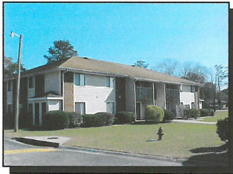
(9) Hillcrest building, Diagonal view.
