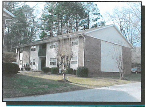
(6) Coleman Street building, southeast to northwest.
