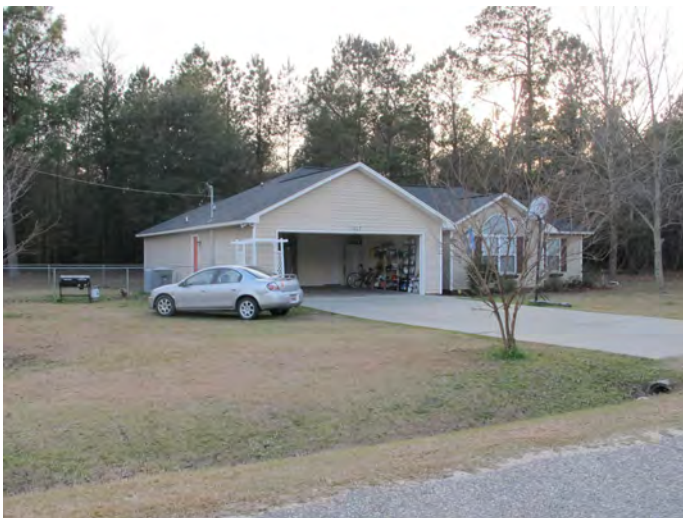
Single-family home located to the Northeast of the Site Manchester Drive.
