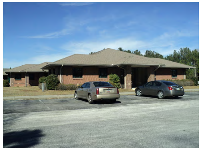
The Department of Mental Health is located adjacent to the Site to the North.
