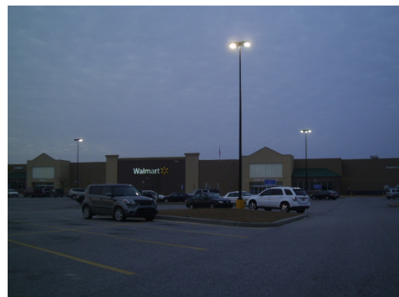
Wal-Mart SuperCenter near site.
