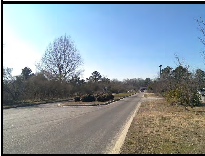
Streetscape west view of Hartsville-Crossing Boulevard
