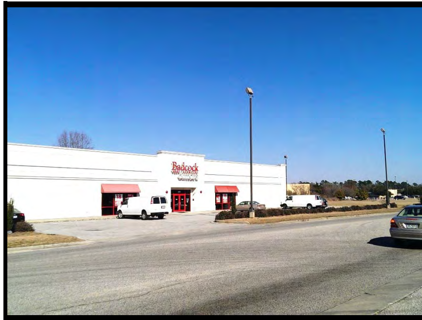
Northeast view from site
