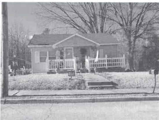
Single family home fronting Gaffney Avenue southeast of site; similar to other homes on Gaffney Ave
