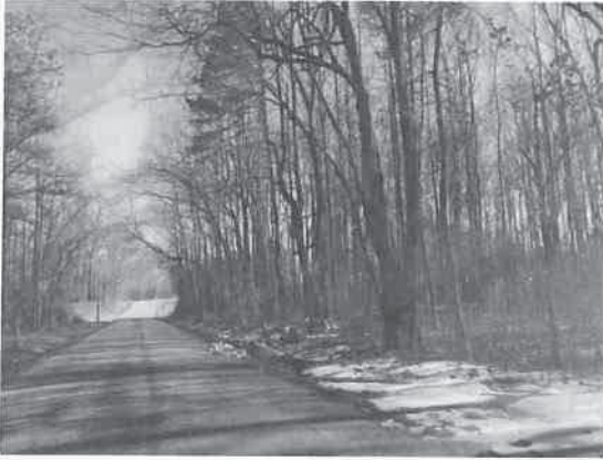
View of eastern boundary of site which fronts Carlisle Street from northeast corner of site facing south
