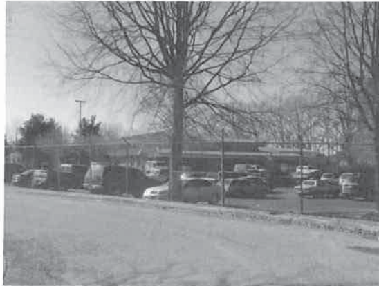
Rear view of US Post Office which is separated from the western boundary of the subject by a wooded lot owned by the US Postal Service
