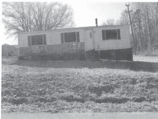
Vacant home adjacent to southeast corner of site; structure to be removed prior to construction of subject
