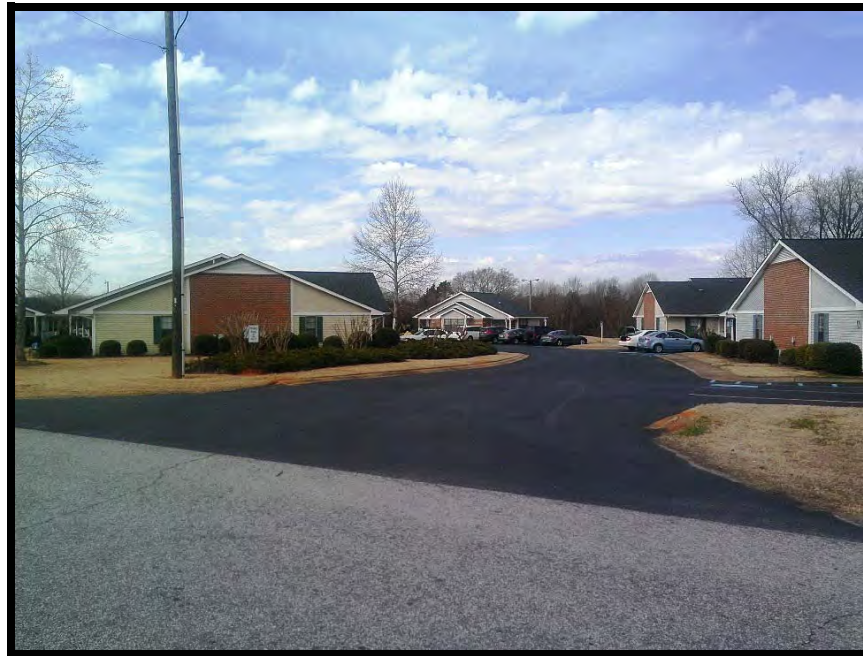
View of site from the southeast
