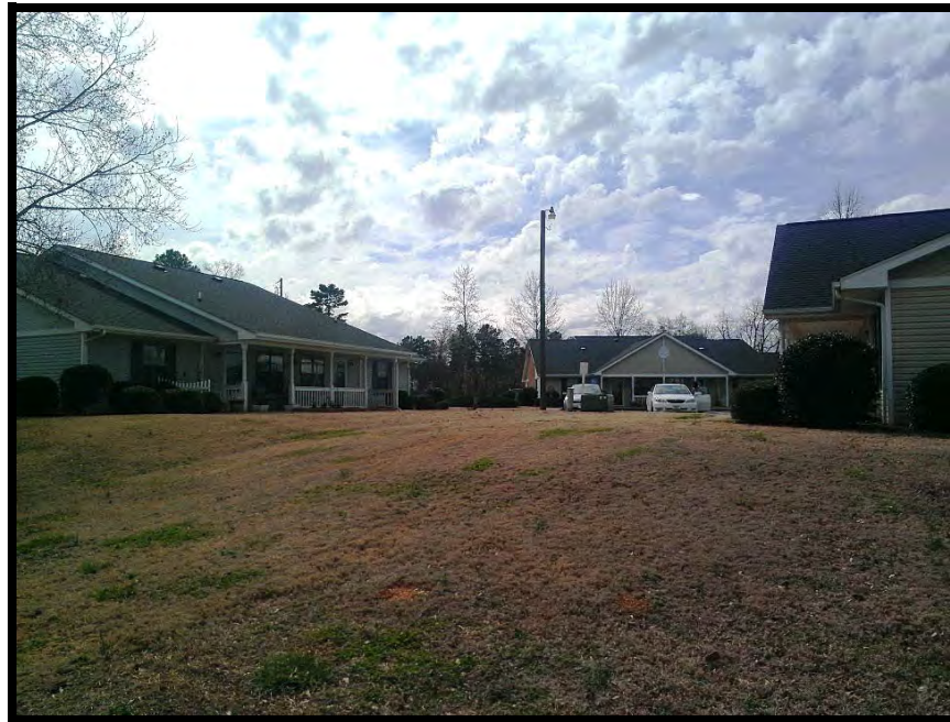
View of site from the northeast
