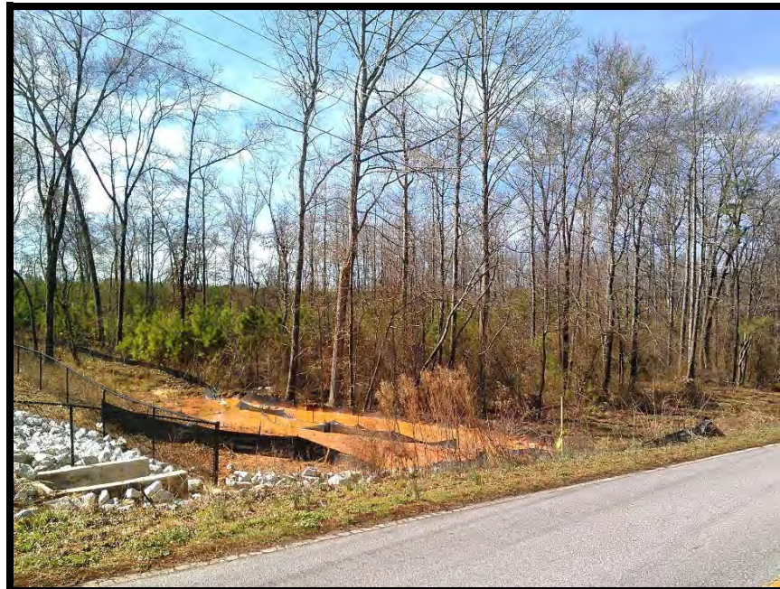
View of site from the southeast
