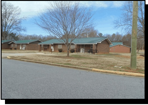
(7) Housing Authority stock, south of site.
