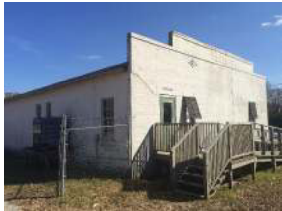
The site and an existing building facing southeast
