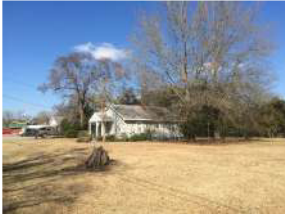
Single-family home bordering the site to the north
