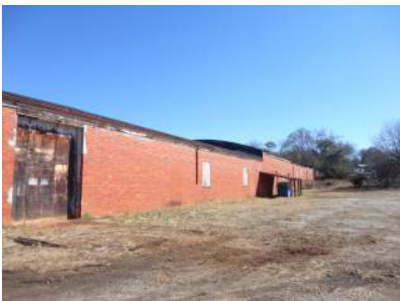
View of existing building on western portion of site.
