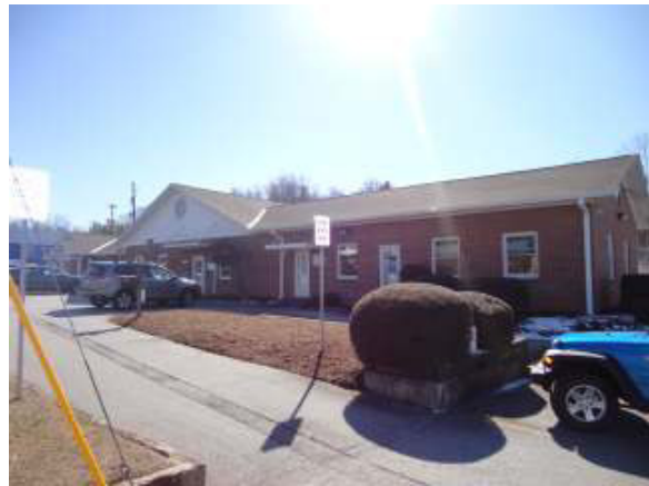
Government building to the west.
