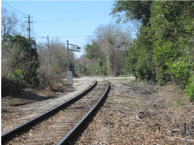
Railroad tracks and crossing northwest of the Subject
