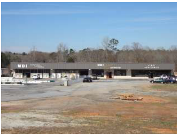
MDI Electrical Plumbing Supply to the south.
