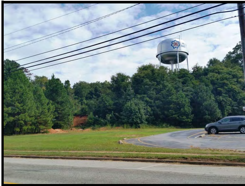
View of site from the southwest
