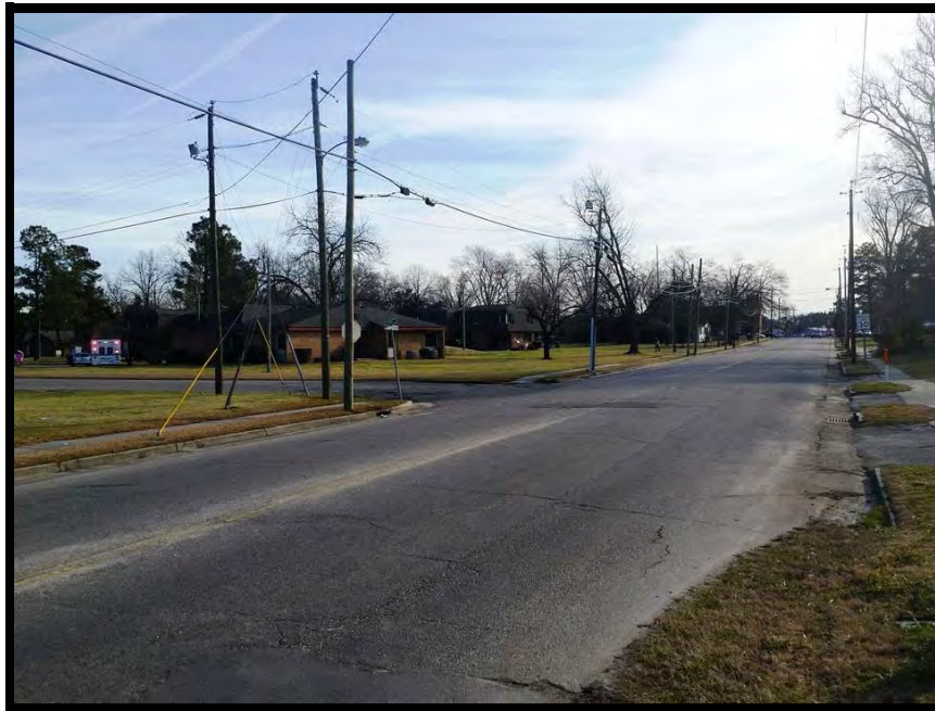
Streetscape: East view of East Godbold Street
