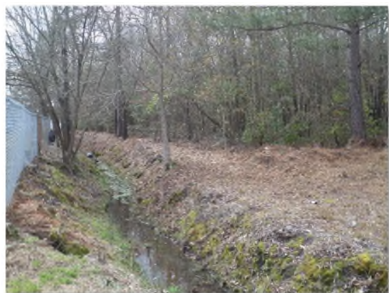
Site facing southwest from behind adjacent apartments on Gertrude Drive.
