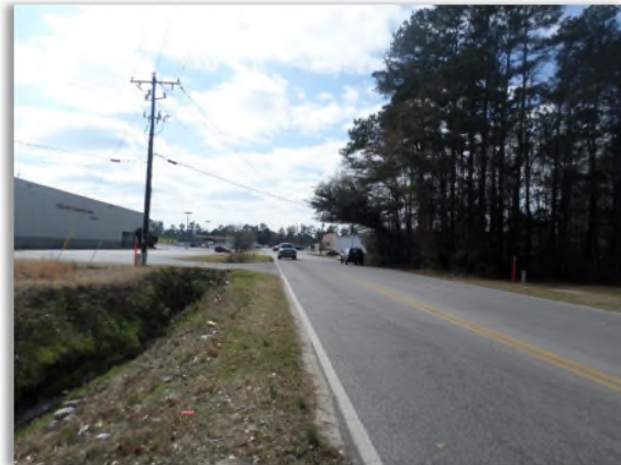
Bultman Drive facing southwest from site.
