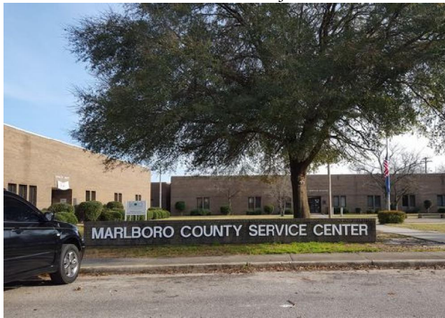
Government offices south of Subject site
