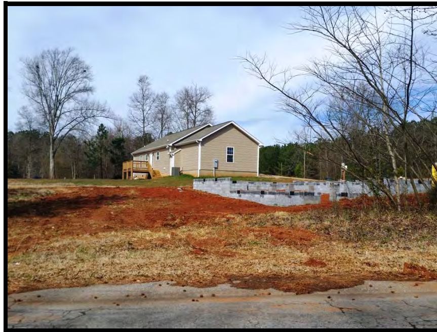
North view from site
