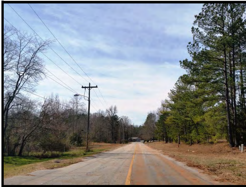
Streetscape: Southwest View on Fairfield Drive
