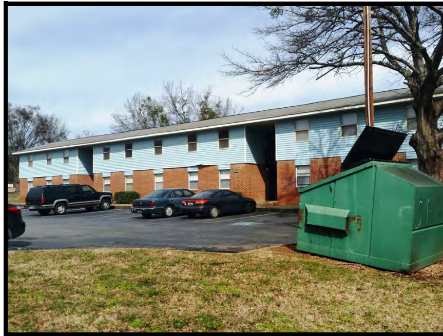
View of site from the southwest
