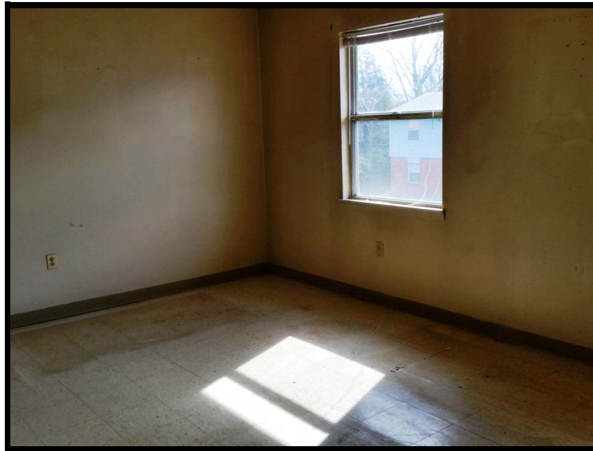
Typical One-Bedroom Apartment Living Room
