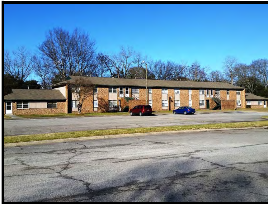
Typical Building Exterior
