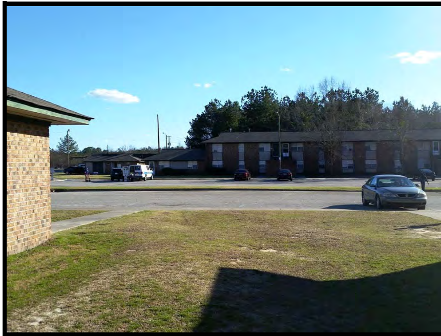
View of site from the north
