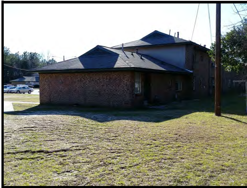
View of site from the northeast
