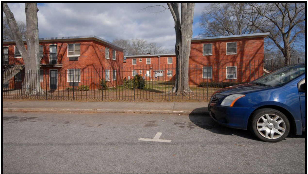
Photo 4—The subject from the corner of Stratham and Crest.
