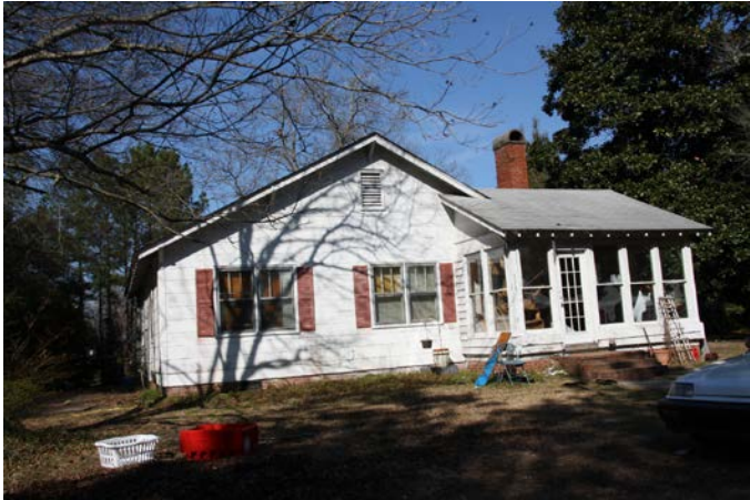
Typical single-family home adjacent to north of site Facing north from Caudle Avenue
