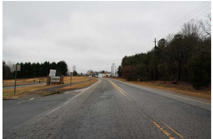
Facing west along Hawkins Road Site is on right School is on left
