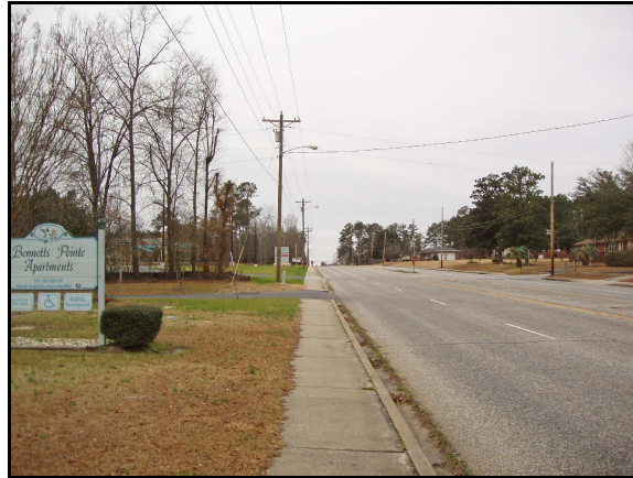
View north on Cheraw St., at site
