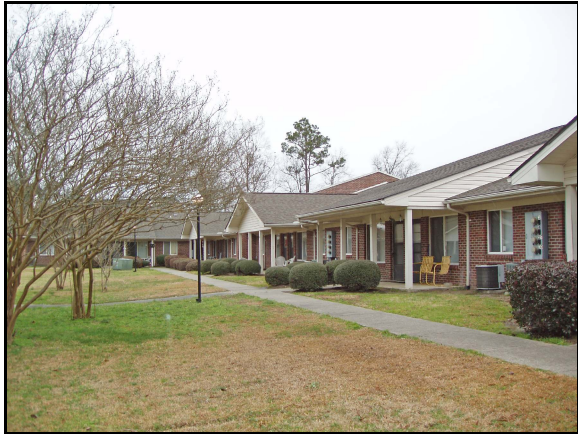
View of typical units, rear of property
