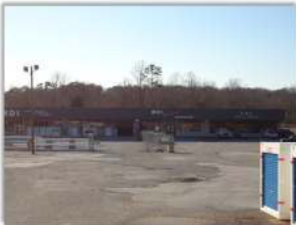
MDI Electrical Plumbing Supply to the south.
