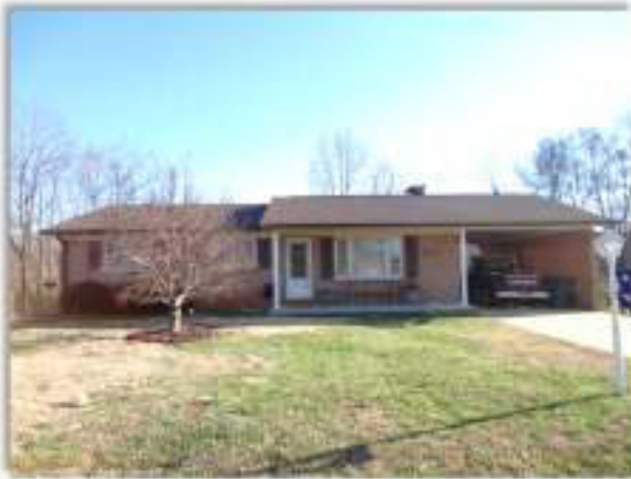
Single-family detached home to the north on Evelyn Drive.
