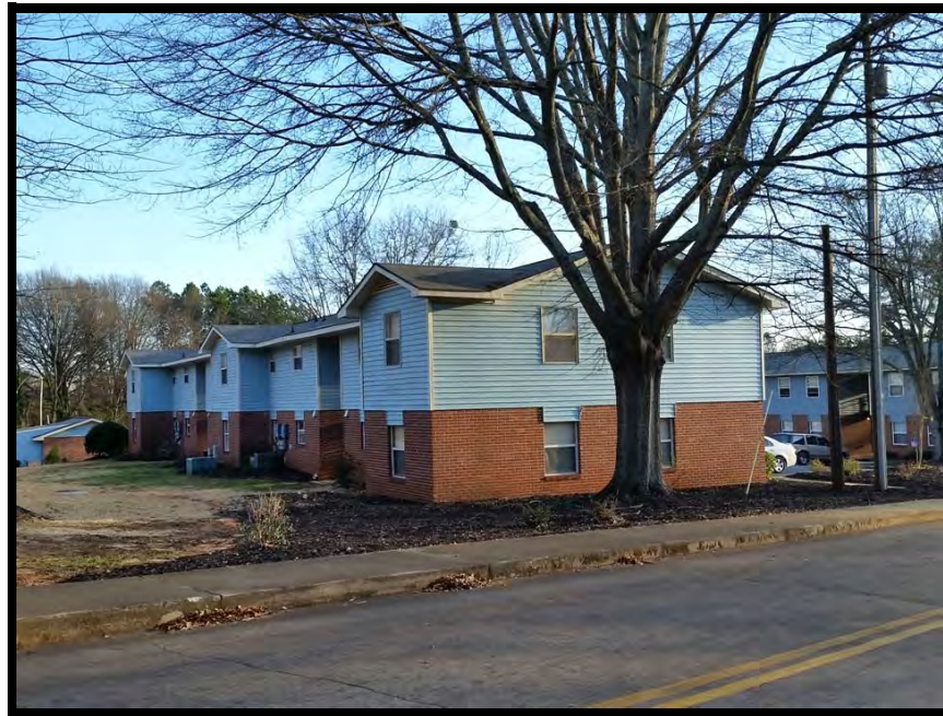
View of site from the northeast
