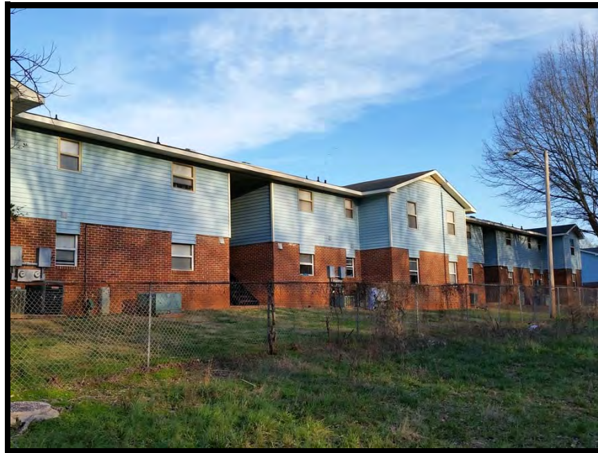
View of site from the west
