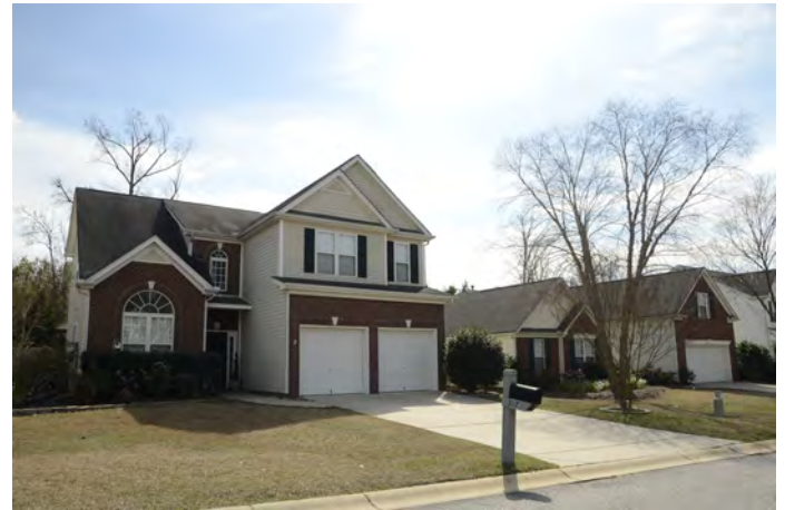
Adjacent Willowbrook subdivision is located on the north side of the Site.
