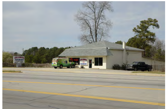
Killman Heating and Air on the south side of the Site at the split of US 1 and US 378.
