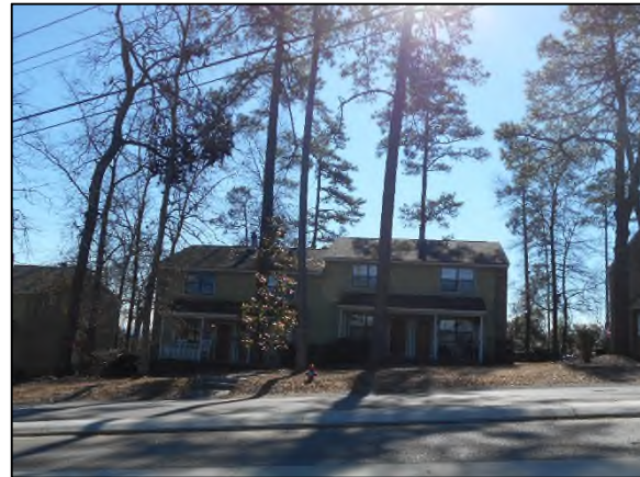
Townhomes to southwest on Lecompte Avenue
