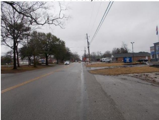
View north on Mill Street
