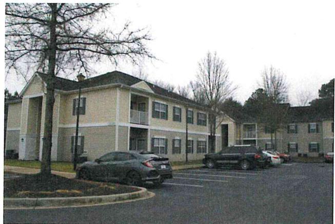
WEST – Apartments adjacent to west of site The Waterway Apartment Homes Facing south from apartment parking lot Site is behind building to left
