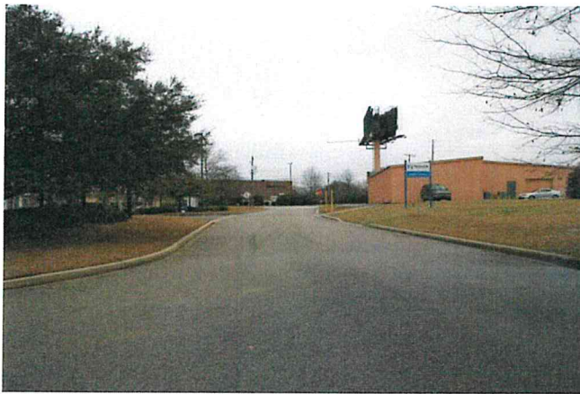
Facing east along Citizens Drive Bank is on left Photo is from site entrance
