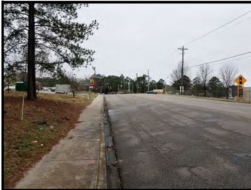
Streetscapes: West view of Brookfield Road
