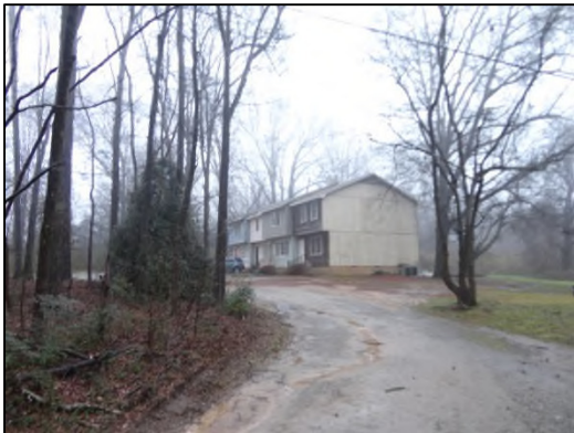
Quadraplex to the north on Shadow Wood Drive.
