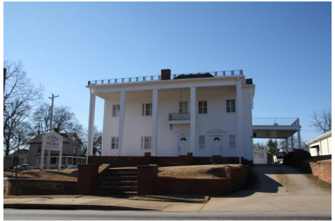
NEIGHBORHOOD – Funeral home adjacent to site Facing southwest from Howard Street
