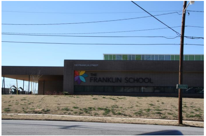
NEIGHBORHOOD – The Franklin School child development center adjacent to the site Facing southwest from Howard Street
