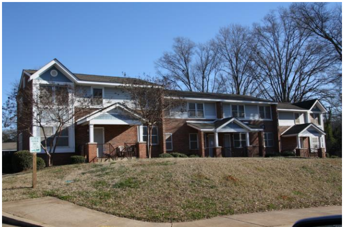
SITE – Victoria Garden 695 Howard Street Spartanburg, SC Typical two-story building
