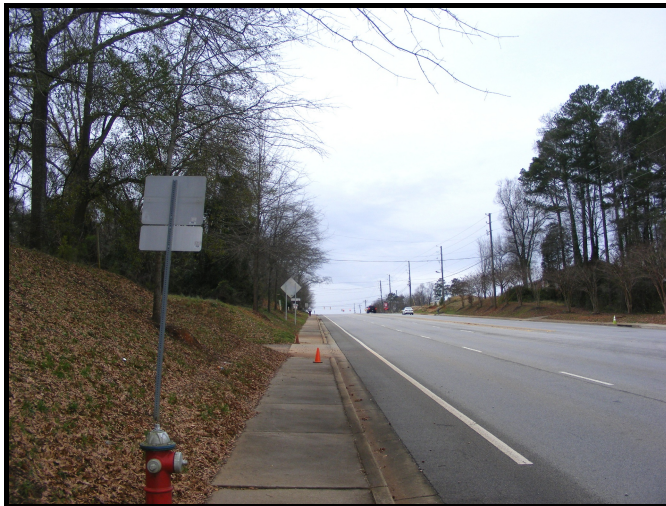
View west on Lake Murray Blvd., at site
