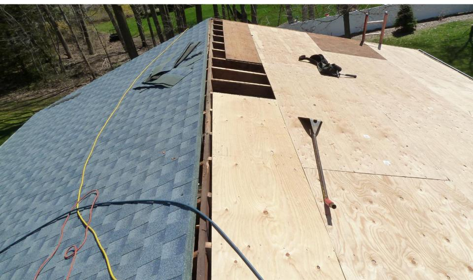
New sheathing, ridge vent cut-in and felt
