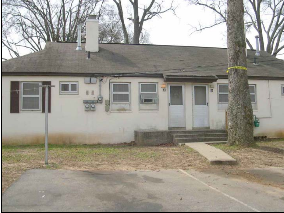
Existing Hub City unit at site
