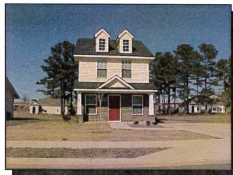
(6) Typical home in Dupont Pointe.
