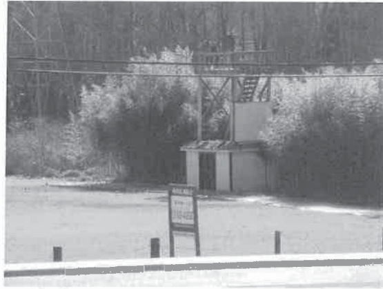
Small wooden structure located in center of site
